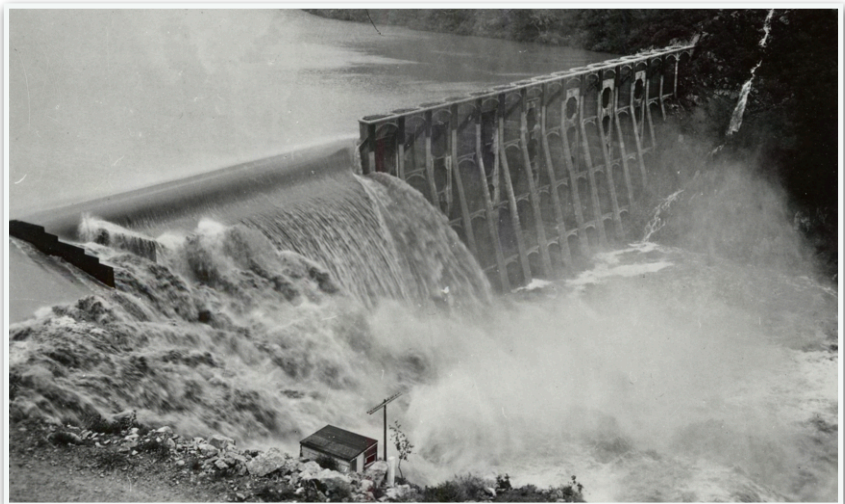
Lake Hodges Dam, completed in 1919. Subsequent construction of a distribution pipe system delivered fresh water to Lockwood Mesa, where the community of La Colonia was created to house workers for area orchards and ranches.
